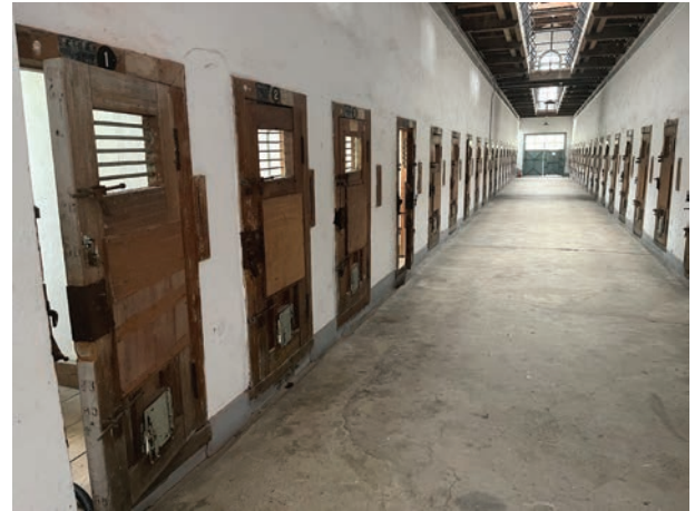
Typical cell blocks with wooden doors.
