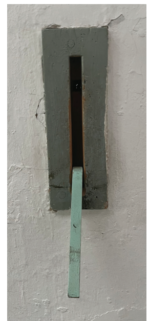
An early form of 'knock-up' button. The wooden lever can be pushed out from inside cells. Prison guards could then physically see the lever was sticking out and investigate.
