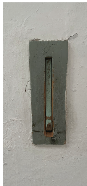
An early form of 'knock-up' button. The wooden lever can be pushed out from inside cells. Prison guards could then physically see the lever was sticking out and investigate.
